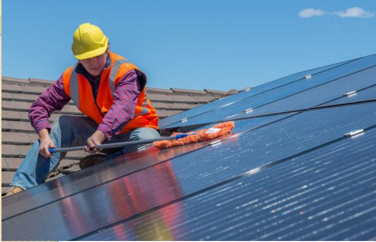
Water-soft cloth wiping
